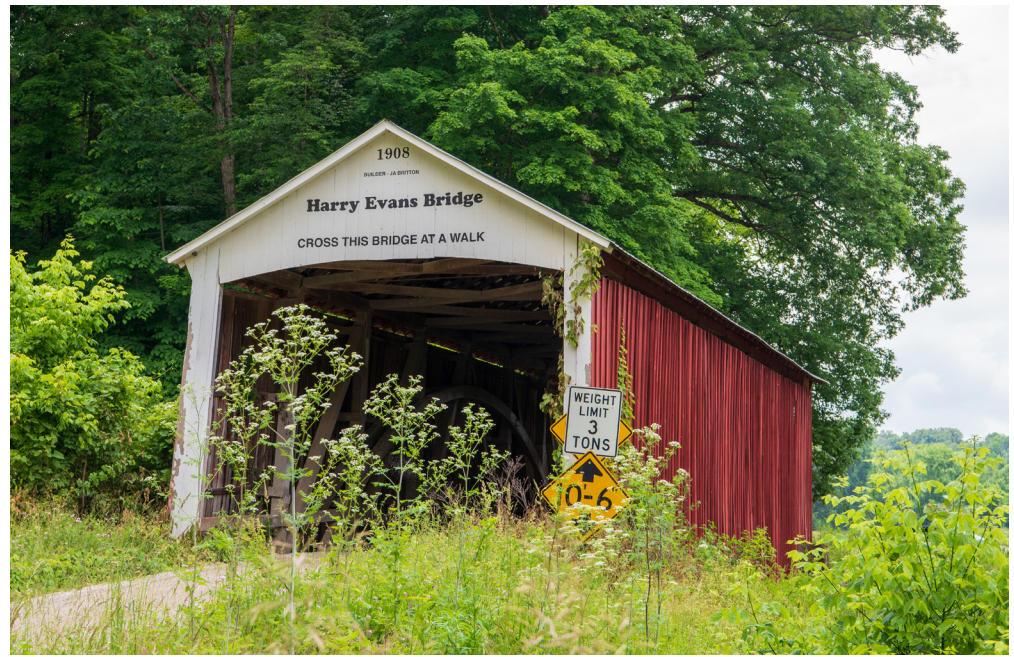
Harry Evans Covered Bridge (#19)
